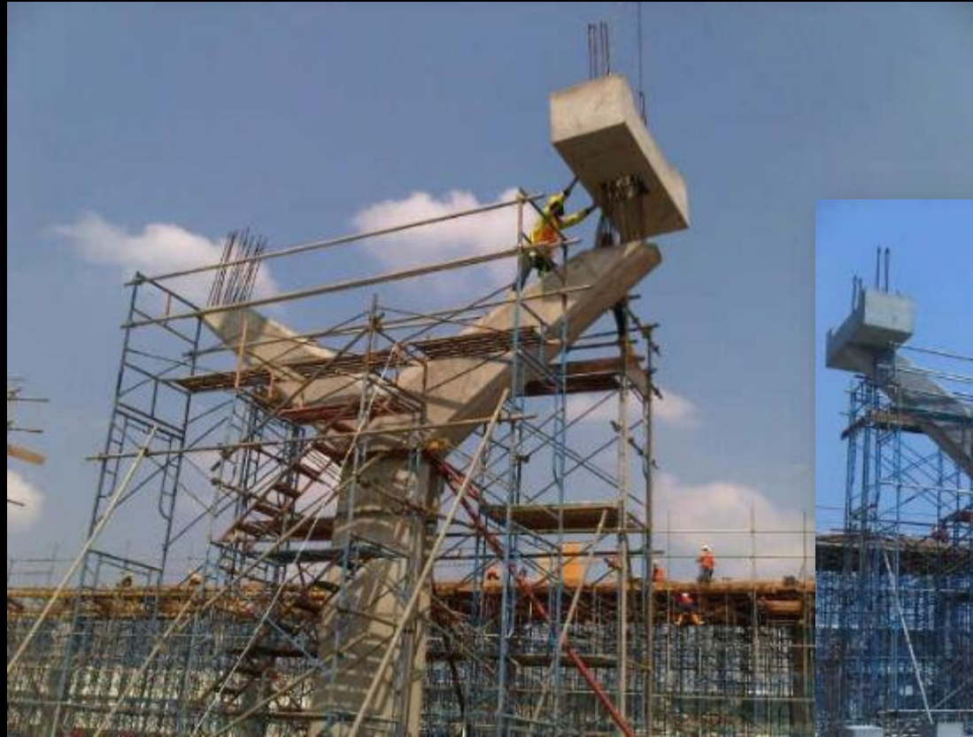
HM Sampoerna - Karawang Beam Column Precast
